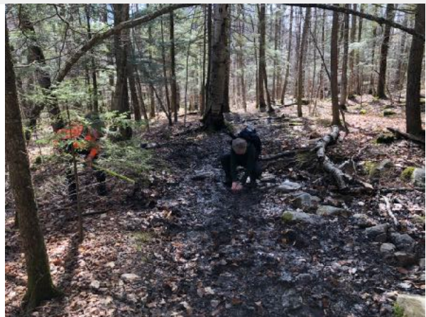
Bald Mountain East Side - water bar work
